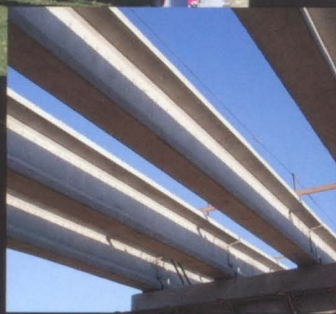
Left: The unfinished overpass looms above motorists.
