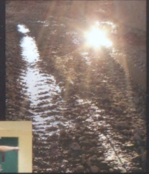
Right: The sun illuminates puddles in the construction area.
